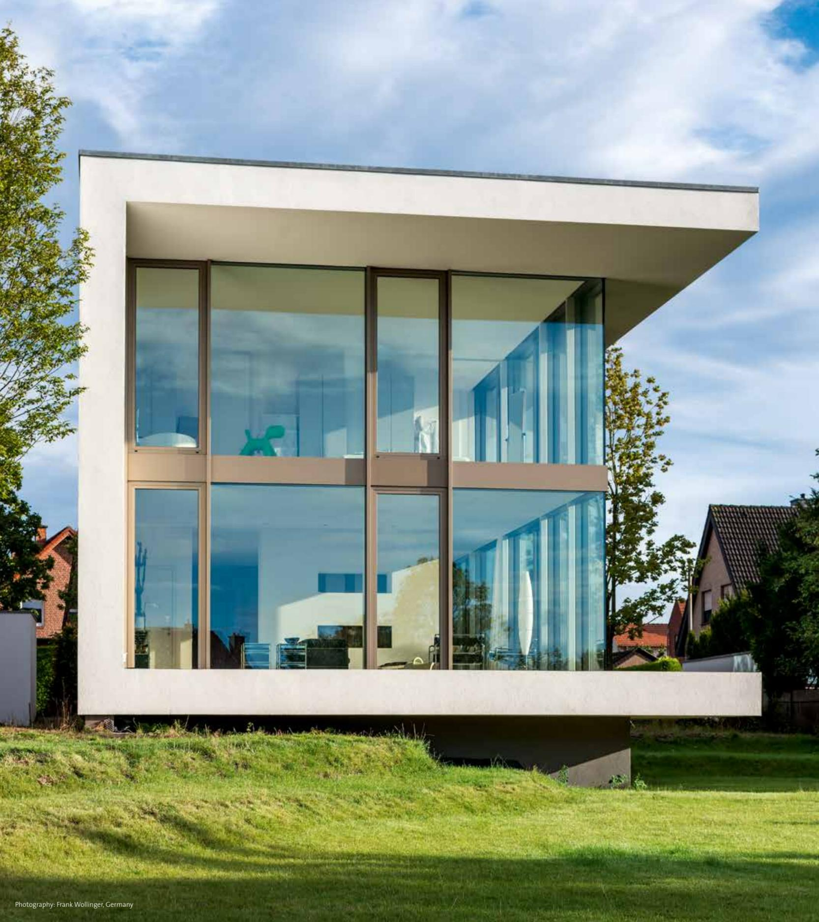
Transparency was ensured by a two-storey high curtain wall with anodised profiles and insert elements.
