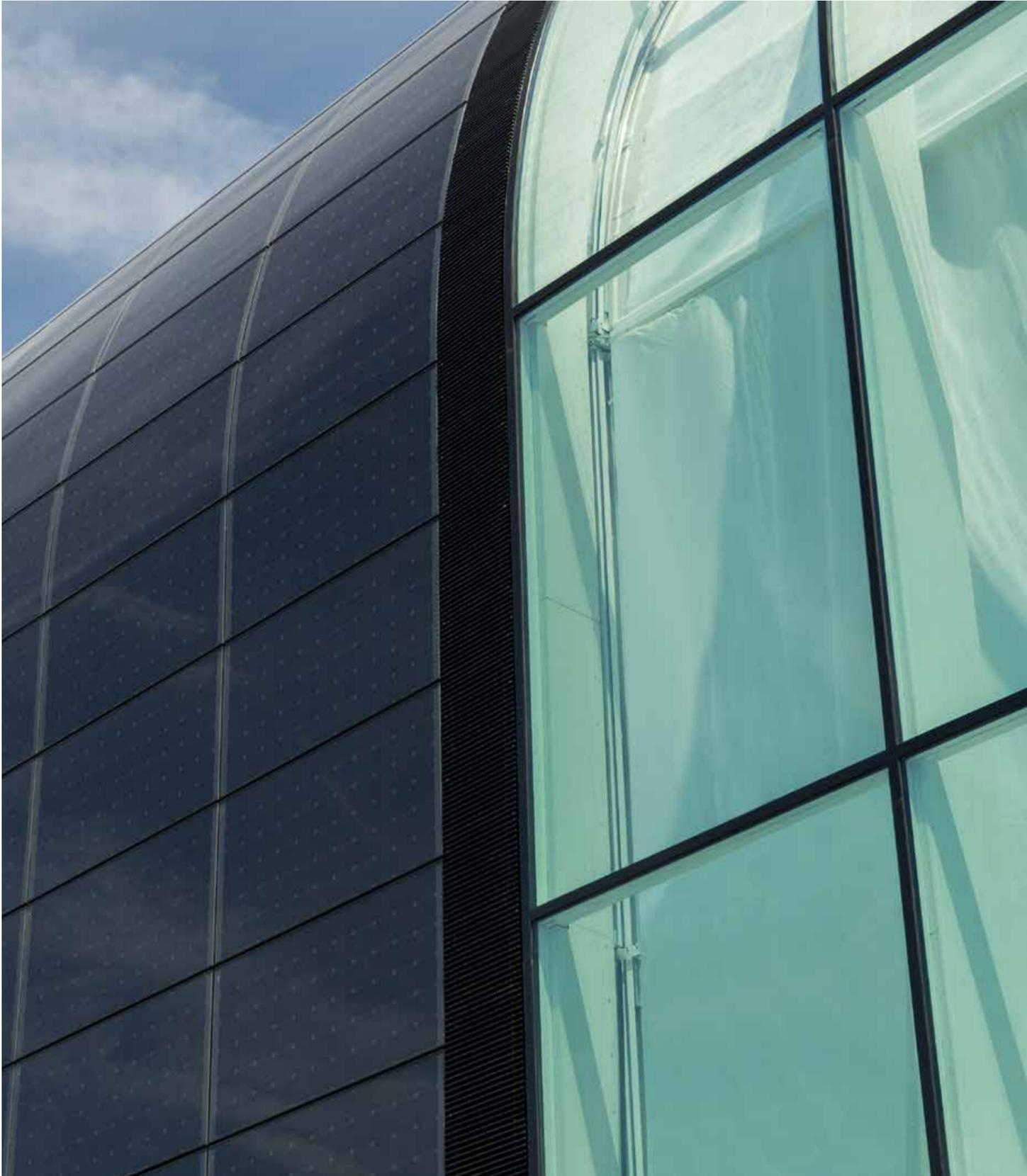
A mix of triple glazing and a unitised curtain wall with outstanding thermal characteristics significantly reduces heat loss via the façade and results in a U-value below  $1.0 \text{ W/m}^2\text{k}$ .
