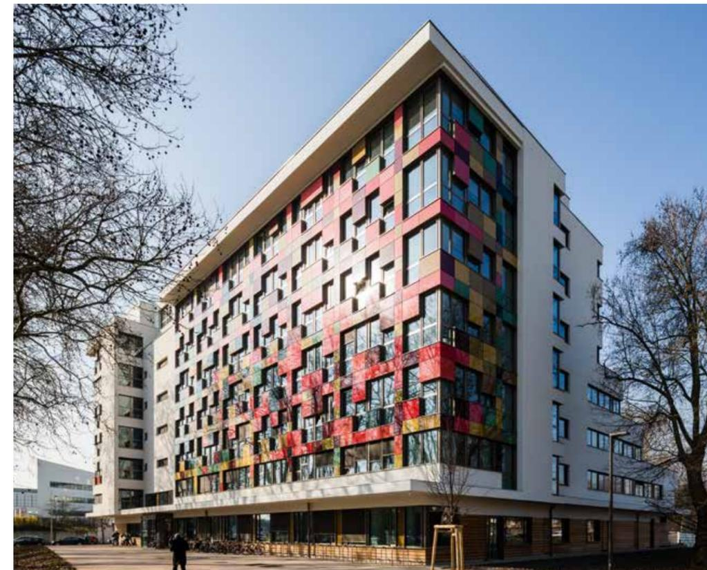
The moving blinds enhance the dynamic colour play of the building. When closed, they shed a soft, dipped light into the office spaces.
