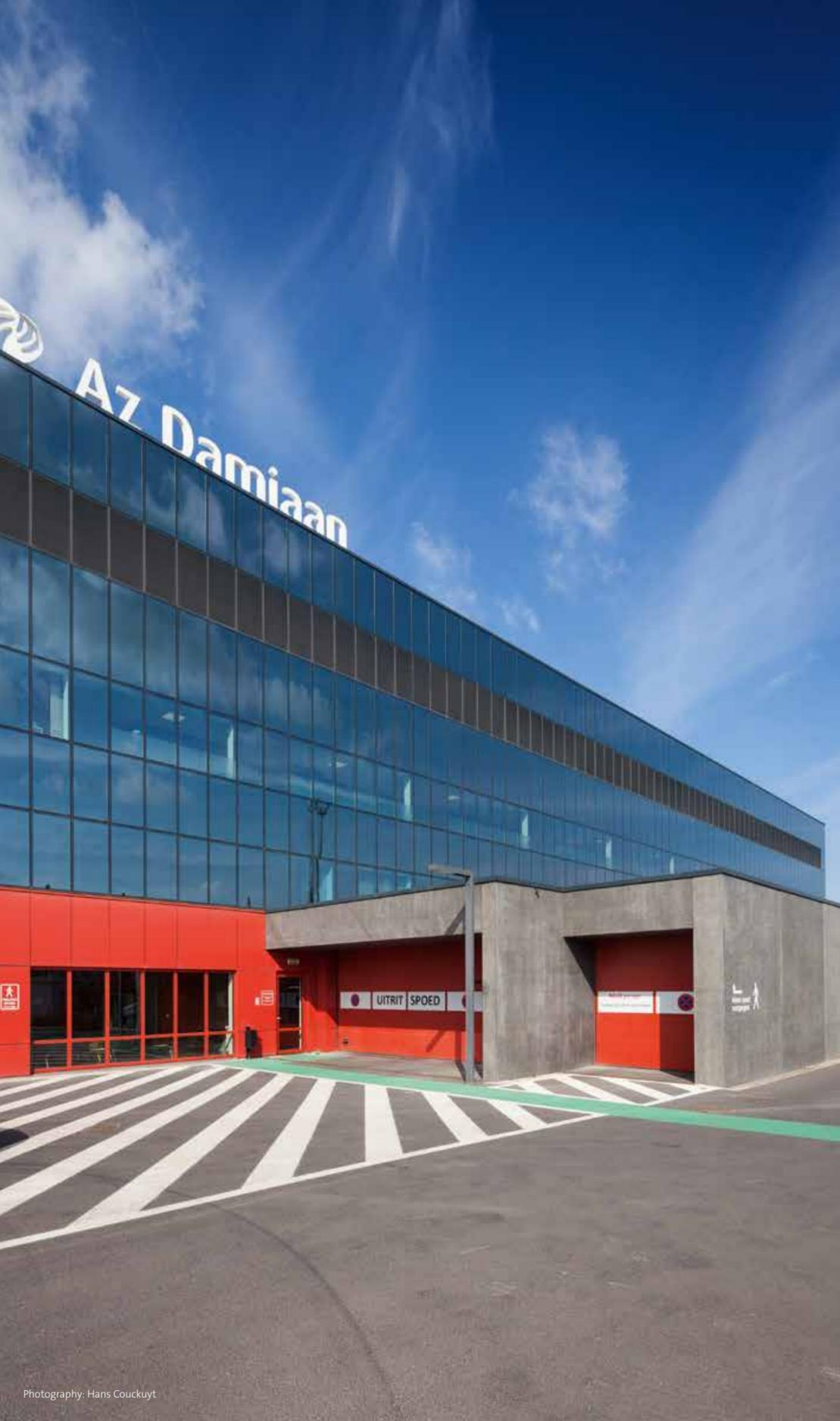
Thanks to Sapa's Confort 125 insulated sliding and lift-sliding system, large areas become easily accessible. The Elegance 52 curtain wall system completes the contemporary building design.
