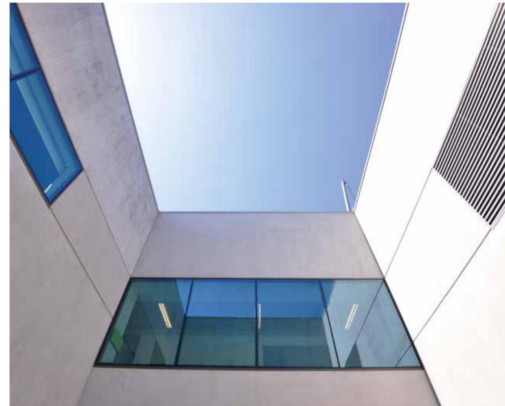
Special aluminium blades ensure that the CMIN building has excellent solar control features.
