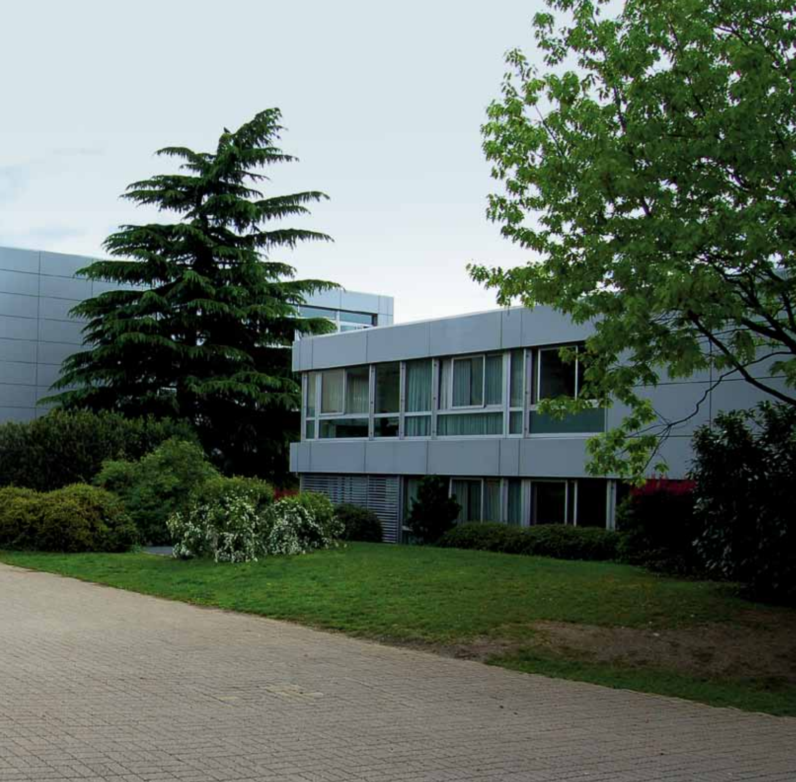
Project: Ecole de Beausorbre City: Morges - Switzerland
